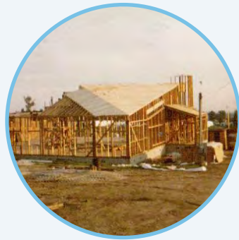
Groundbreaking of current building
